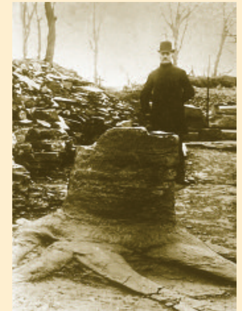
Above: Fossil Grove after excavation of the tree stumps prior to the construction of the building around them (late 1880s).
